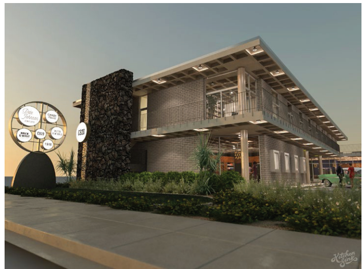
This latest adaptive reuse project from Wetta Ventures and Brick & West Design takes a conventional midcentury office complex in Phoenix, and reimagines it for the present and future, producing a retro-contemporary mixed-use complex, soon to be anchored by exciting entertainment venues with daily-use creative office space above.
